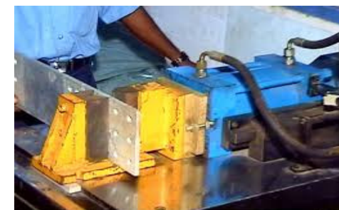
HYDRAULIC BUS BAR BENDING
